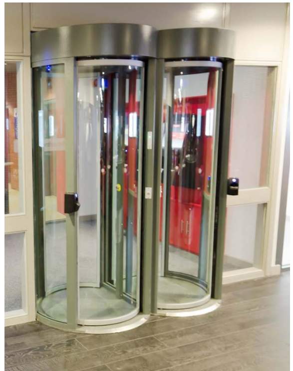
TWIN TONDA WITH BIOMETRIC READER ACCESS CONTROL
